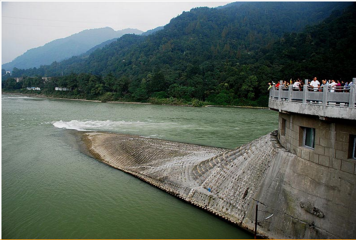
Fish Mouth Levee - Irrigation head at Dujiangyan Irrigation System in China.
